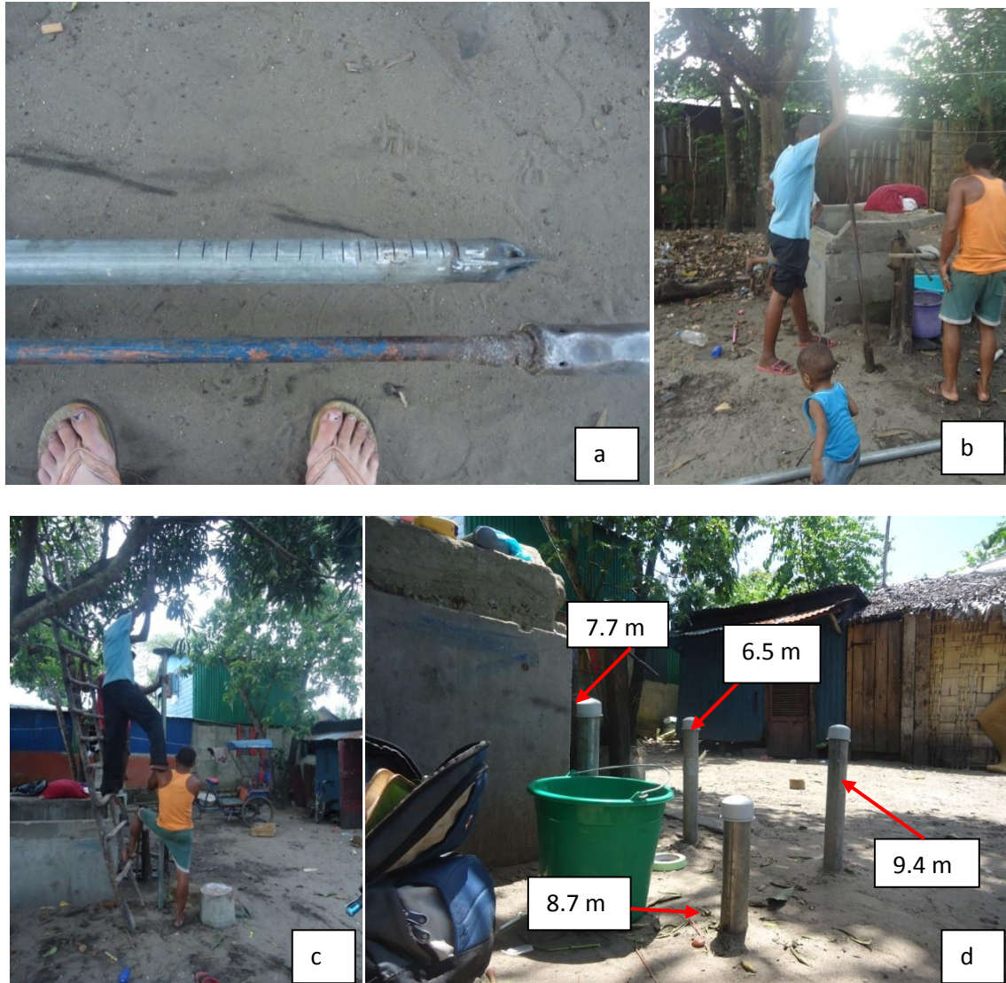
Figure 13: Materials and processes used to install the monitoring wells. (a) The GI outer casing (top) and agar(bottom) (picture taken by the author); (b) The technician's assistant drilling down near the water table (picture taken by the author); (c) The technician hammering the well into place (picture taken by the author); (d) Four completed monitoring wells with their corresponding depths noted (picture taken by the author).
