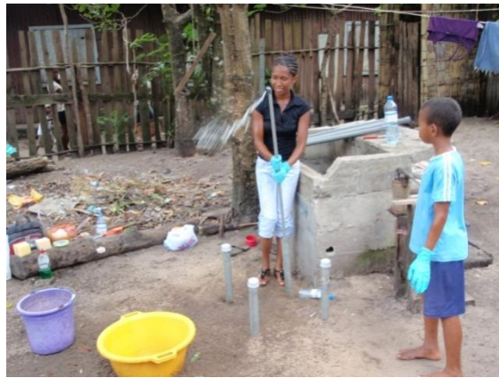
Figure 14: The Malagasy research assistant developing the monitoring wells. Development was done using a technique based on EMAS methods (picture taken by Michael MacCarthy).
